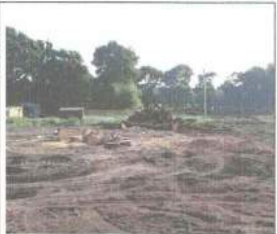
Photograph 2 – The southern aspect of the site
