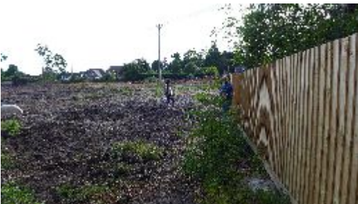
B: VIEW INSIDE THE SITE: SOUTH WEST
