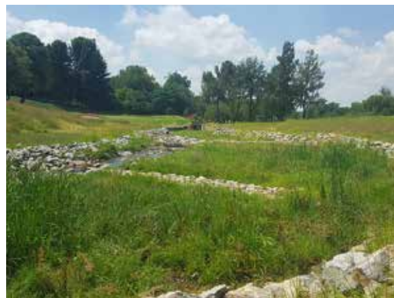
Dry attenuation basin
