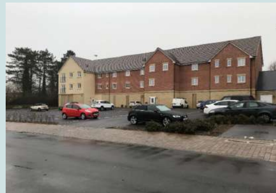
› Rear view of Block C with parking court.
