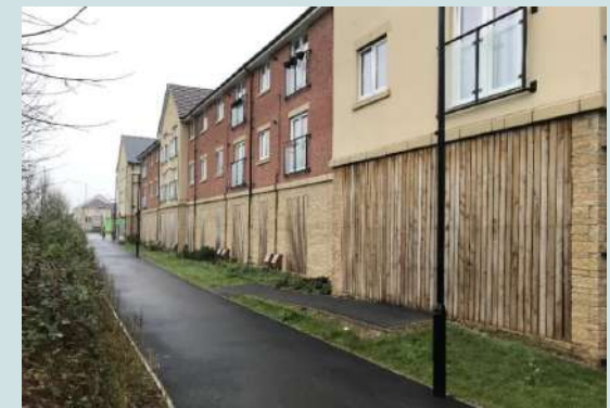
› Front elevation of Block C.
