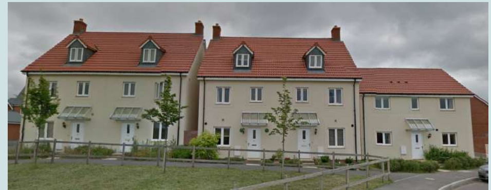
› Existing 2.5 storey render dwellings at key space on Roger Way..
