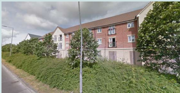
› View of Block C from Portway.
