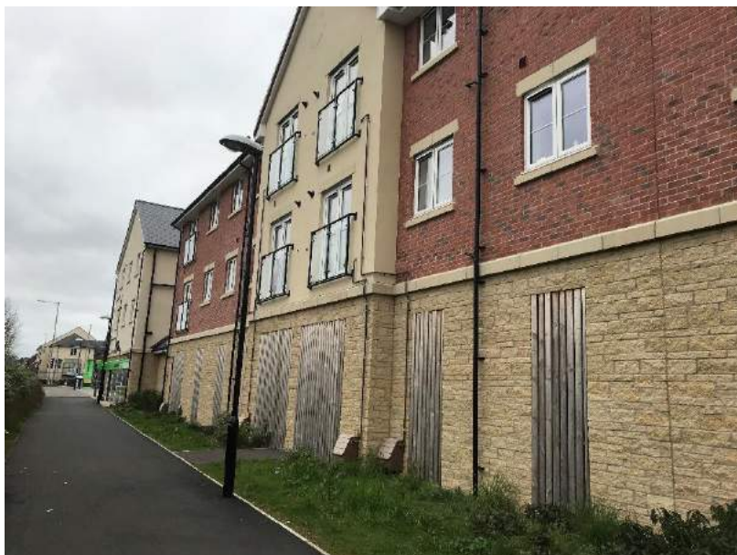
Photograph 1: View of buildings in land parcel G; south-east elevation.
