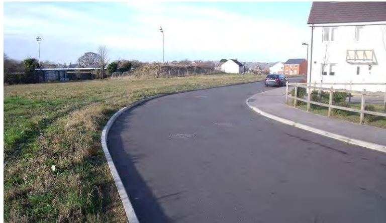
Photograph 2.1: Roger Way (Looking North) showing main development site
